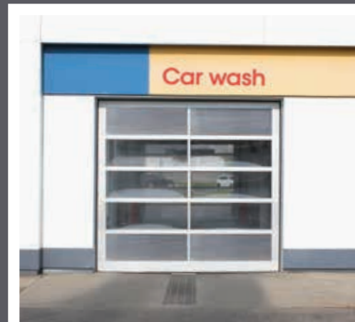
Multiwalled polycarbonate 5/8" (16 mm) thick. Polycarbonate units are available in three colors: clear, dark bronze or opal.
