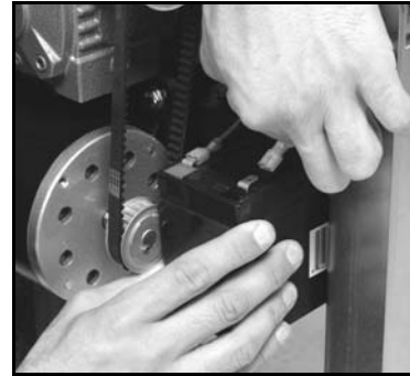
Reconnect the wires onto the replacement batteries.
